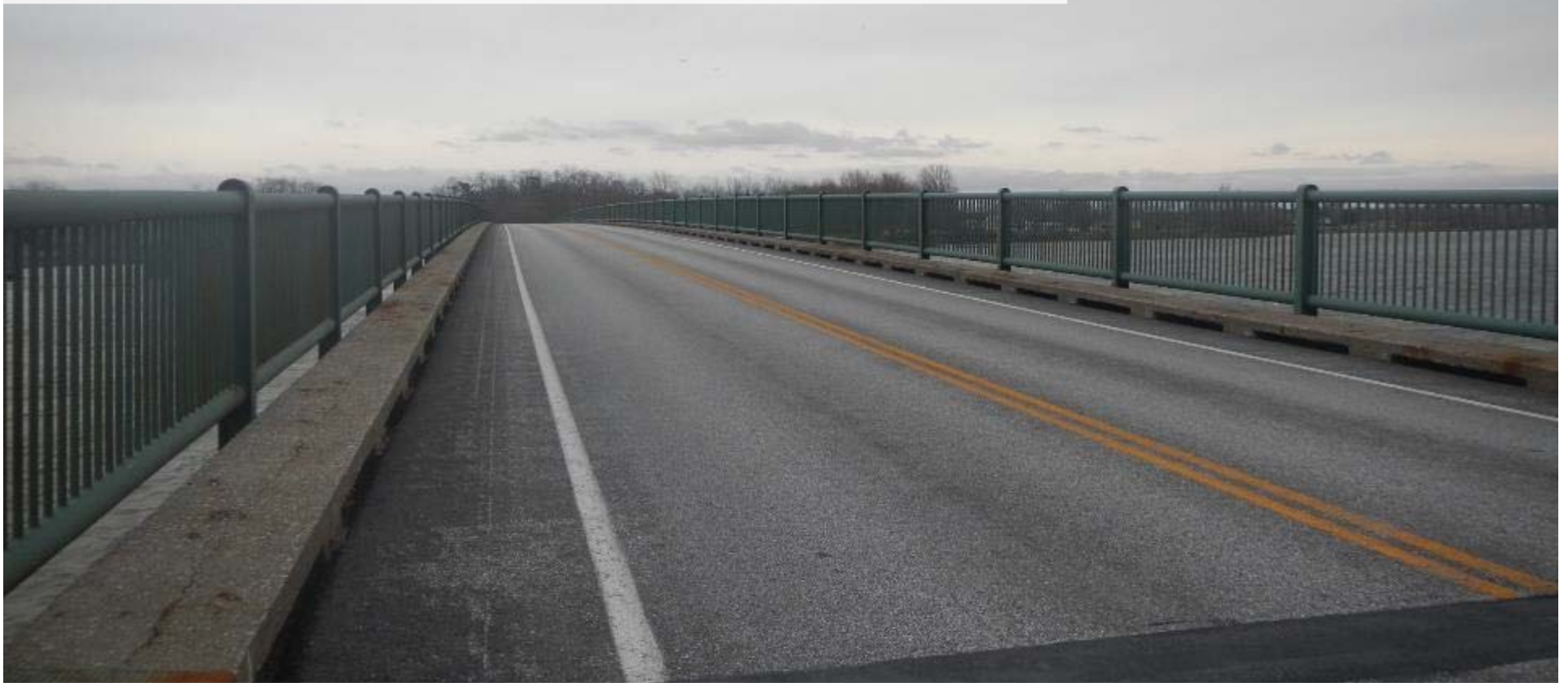
Typical Top of Deck Condition
